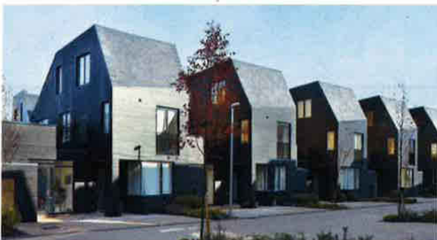
Innovative housing types at Newhall, Harlow
